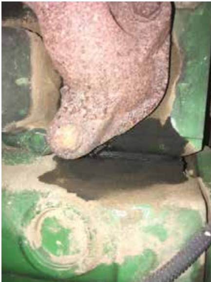
There is an engine oil leak in this head gasket which will need to be addressed.
